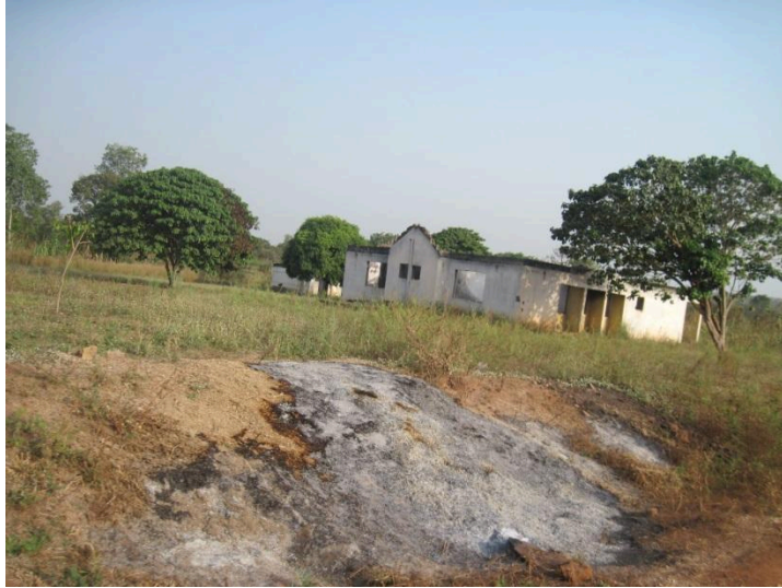
Remains of a destroyed property near Kaseyo
